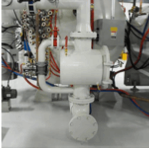
Water-cooled binder trap assembly
